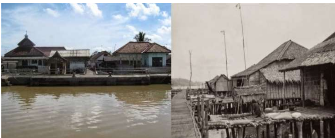
Figure 3. House Shape at Kampung Laut in 1935 (right) and at present (left)
